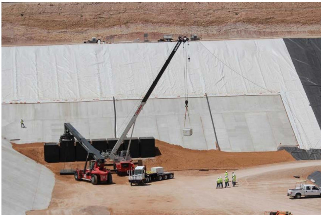
Figure F-21 Wastes being Loaded into Rectangular MCCs inside a Disposal Cell with Components of the Multi-Barrier Liner Visible in the Background (Note the scale of the disposal cell.)
